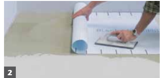
2 Apply Blanke•SECUMAT to the substrate and embed mat with float or roller. *NOTE: Observe open time of chosen mortar.
