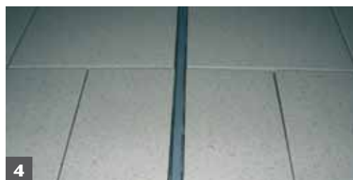
4 Remember to install perimeter joints and Blanke expansion joints per TCNA guidelines EJ171. *NOTE: Read complete instructions before installing.
