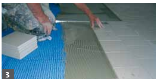
3 Work thin-set mortar into the surface of Blanke•PERMAT and set the tiles.
