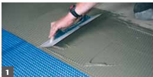
1 Apply loosely mixed modified thinset to the substrate using a 1/4" x 1/4" notched trowel.
