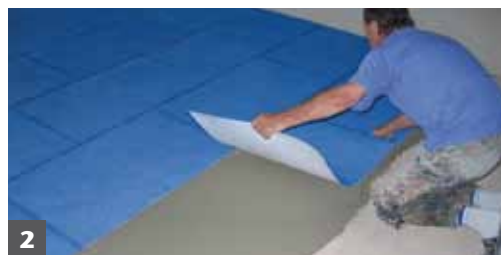
2 Install Blanke•PERMAT fleece-side down, making sure to overlap and keep 3" min. offset pattern. *NOTE: Observe open time of chosen mortar.
