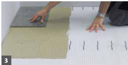
3 Work thin-set mortar into the surface of Blanke•SECUMAT and set the tiles.
